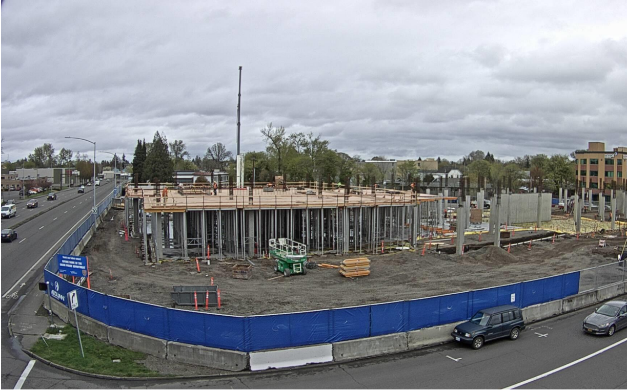
View From Police Station Project Cam – April 11, 2019
